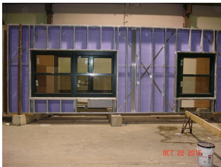
A completed wall segment ready for shipment.
