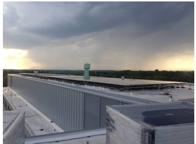
Solar Panels atop of Kasych Pavilion
