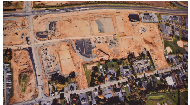
Aerial view of site
