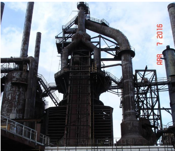
Feeding the furnace. Note the dual "tracks" in the middle of this picture that lift the "skips" to the top of the furnace.
