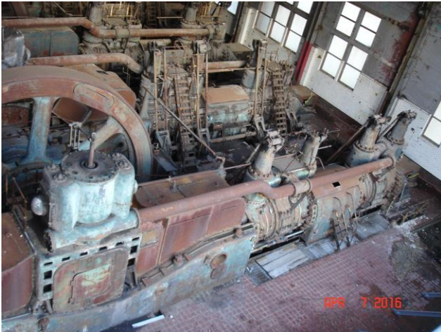
Air compressors for the blast furnaces.
