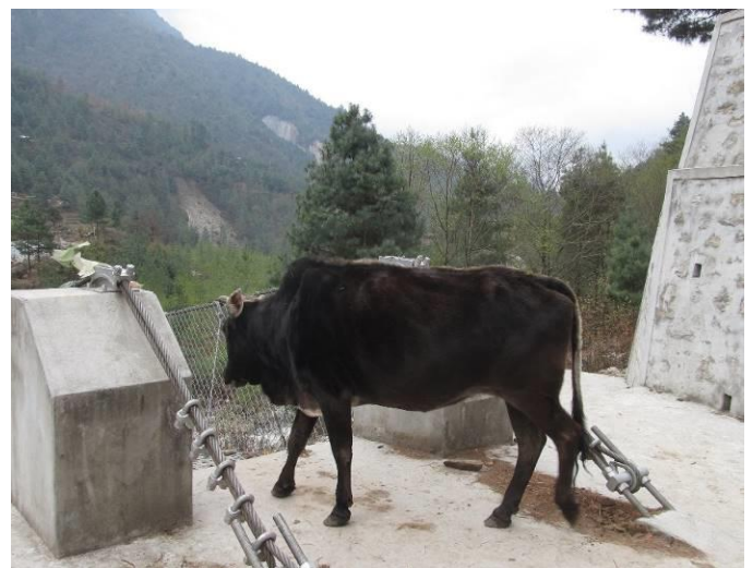
Note anchoring system. In times past, vines were used instead of steel cables.
