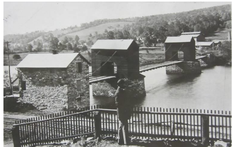
Lehigh Gap Chain Link Bridge, early 20 th Century. Note the single strand chain. Photo courtesy of Chad Schwartz, Director of Science & Education Lehigh Gap Nature Center, Slatington, PA.
