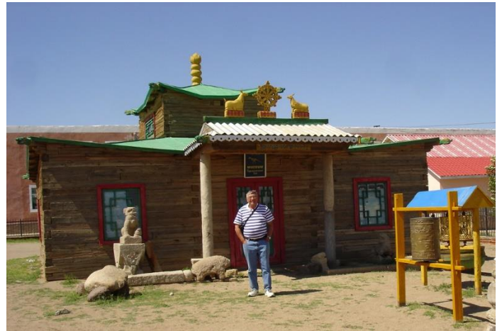
A Buddhist temple. The building is built with 4" x 4" wooden beams. Note the prayer wheel on the right.
