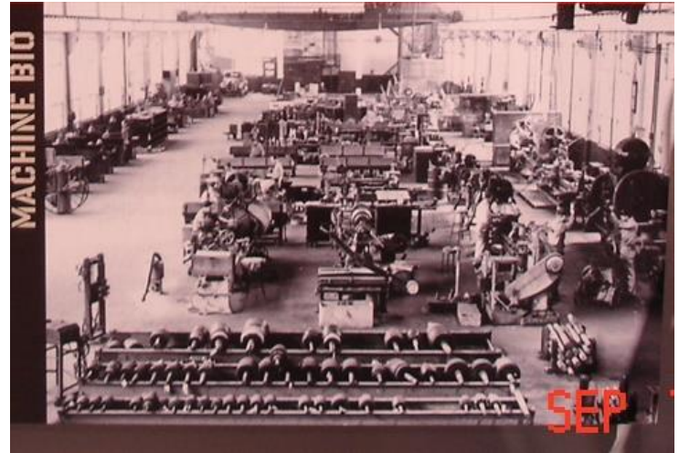
Floor of the electrical repair shop
