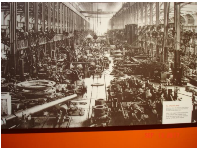
No. 2 Machine Shop
