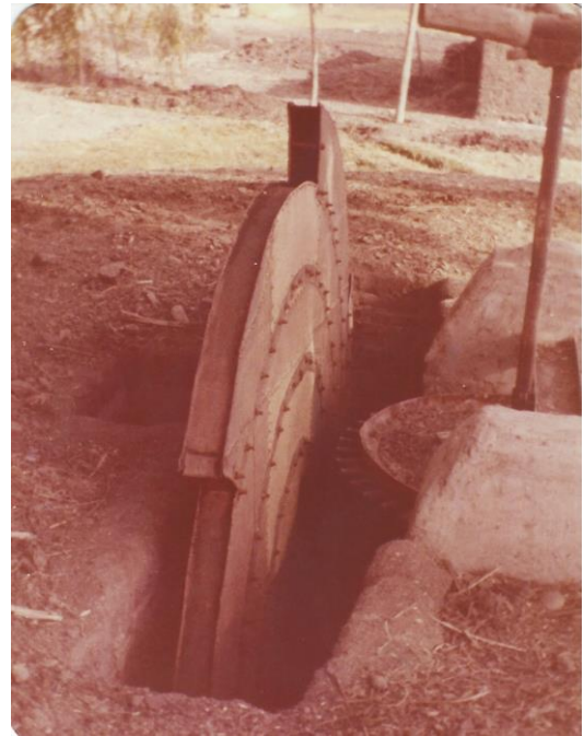
A water wheel, to raise the water to a higher level.
