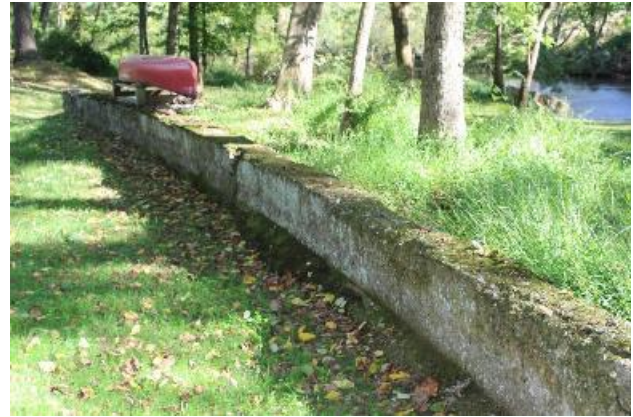
Vestiges of the Erhart Grist Mill millrace. Note Saucon Creek on the right. This is on private property.
