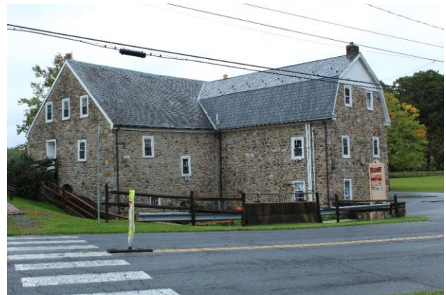
Mill building. Water enters the building on the left.
