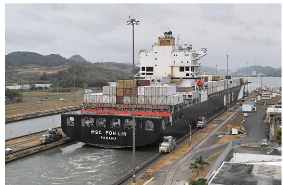
Gatun Lake provides the water to raise and lower vessels in the Canal, gravity fed into each set of locks
