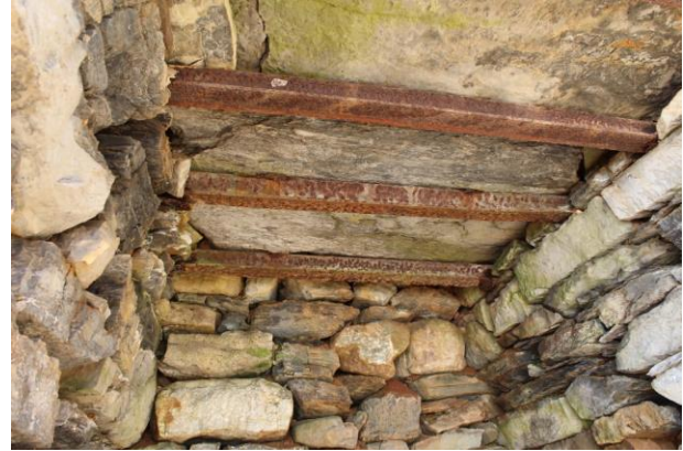
Lime kiln along Lime Kiln Road. Note rails on top of chamber.
