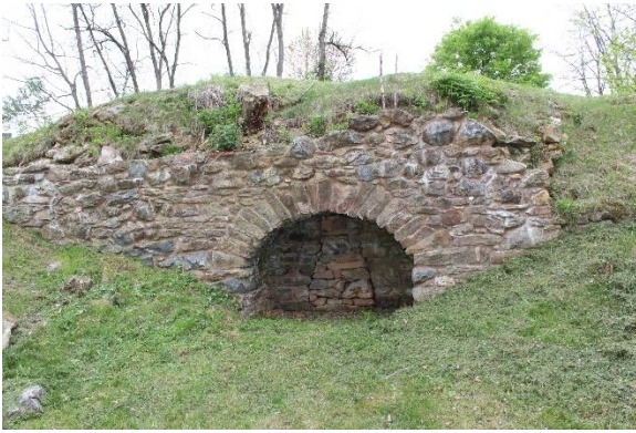
Springtown lime kiln. The opening is 6' wide by 5' high. Note the bottle-shaped opening in the rear. The shape of the rear opening is similar to other lime kilns in the area.
