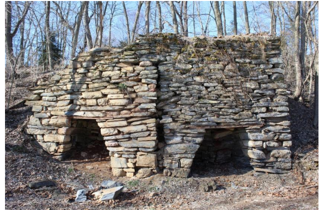
Two kilns along River Road. They are approximately 4' x 4'. Again, the limestone quarry is next to the kilns.
