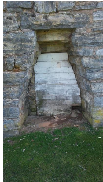
4' x 6' lime kiln, adjacent to the quarry and #15 green. It is boarded up.
