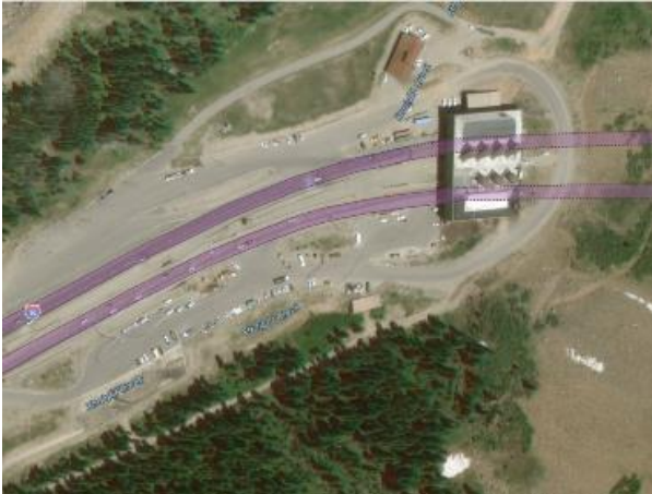
West end of Eisenhower tunnel, with Straight Creek flowing west.
