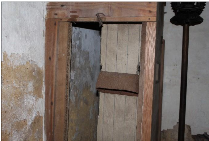
"Down" side of a bucket elevator. The buckets are approximately 6" wide.
