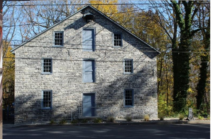
Helfrich Springs Grist Mill. Note hoist attachment above the three blue doors.
